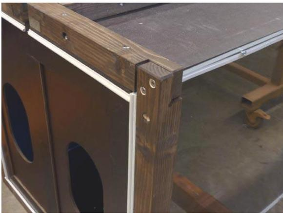
The end girder of the cross-duct modules were equipped with band seals in order to make joints waterproof.
