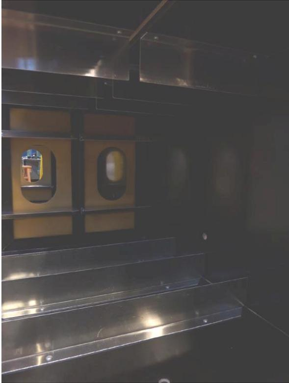
Inside view of a cross-duct compartment with stiffeners attached to the bed, roof and girders.
