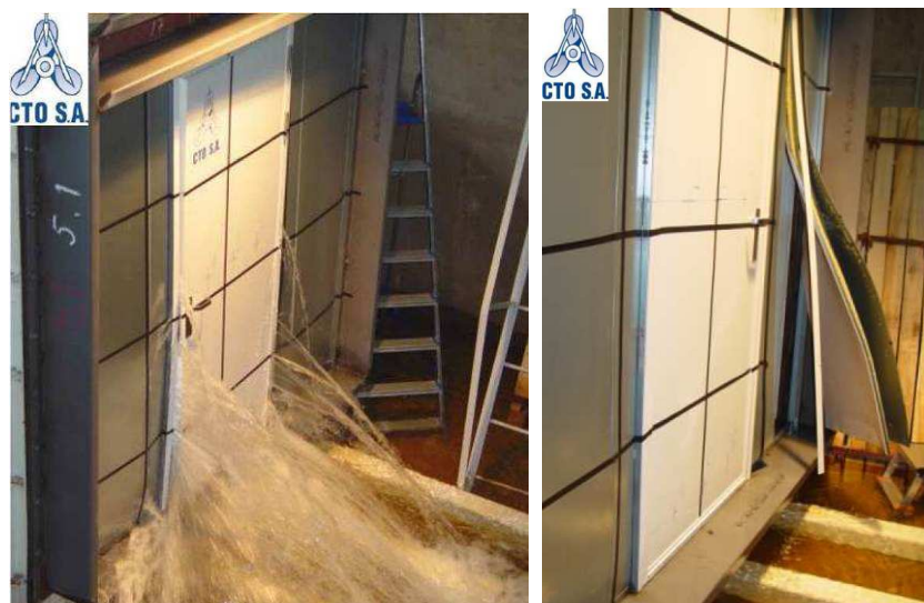
Figure 14: Leakage of a B-class joiner door under 11.9 kPa pressure into the doorframe (left) and damage to the wall panels when the pressure direction was the opposite (right)
